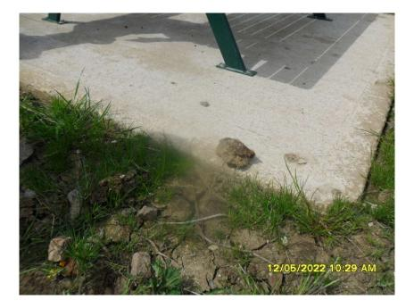
5-Apply topsoil to take out trip hazard between concrete bases and grass area, pic below.
