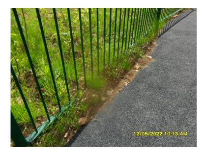
1-Rubber safety surface should be laid in one pour, there are visible joins in the safety surface which are separating and will only get worse over time. This is not acceptable.
